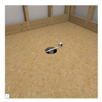
Cut the DN50 pipe even and flush with the subfloor surface. Make sure that the cut out fits to the Fundo base's drain. Cut out a 130 mm diameter hole around the DN50 pipe's center to allow for the wedi drain to be inserted into the subfloor while the cut out area must remain free of deflection. The drain waste pipe and P-trap have to be safely affixed to and supported by the subfloor structure.
