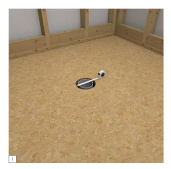
Cut the DN80 or DN100 pipe even and flush with the subfloor surface. Make sure that the cut out fits to the Fundo base's drain. Cut out a 130 mm diameter hole around the pipe's center to allow for the wedi drain to be inserted into the subfloor while the cut out area must remain free of deflection. The drain waste pipe and P-trap have to be safely affixed to and supported by the subfloor structure.
