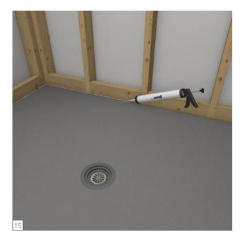
Set up a continuous 10 mm bead of wedi 610 adhesive sealant along the pans channel on the outer perimeter and only in areas where you can immediately install a building board into the fresh sealant.
