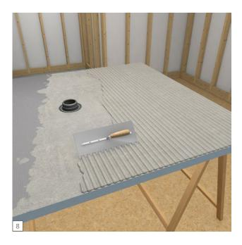
Trowel the tile adhesive on the rear side of the Fundo again using a  $10 \times 10$  mm notch trowel. There are different ways to ensure good bond of the wedi base to the subfloor. Applying tile adhesive on both, wedi base and subfloor, is a best practice recommended to achieve full surface coverage adhesion.
