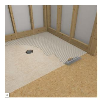
Trowel the tile adhesive and comb through with a 10  $\times$  10 mm notch trowel. Channels pointing to the entrance.
