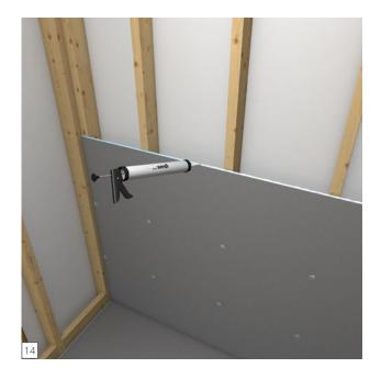
Push the wedi board all the way into the channel of the shower base channel and its bead of sealant. Smooth out any pushed out sealant on inside seam using a putty knife. Fasten the boards directly to the studs starting 300 mm above the base and at a rate of 1 fastener per 300 mm. One extra fastener is set into the seam to the next board to create a flush transition.
