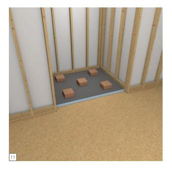
Press the Fundo firmly into the tile adhesive bed, ensuring that the installation is level and void free. Apply some weight equally and leave on surface and drain area to allow the tile adhesive to initially cure without being disturbed (e.g. tile adhesive bags). Do NOT step on the drain module to push/connect to drain body or tile adhesive. Ensure there is 100 % tile adhesive supporting the drain channel area over a completely flat subfloor
