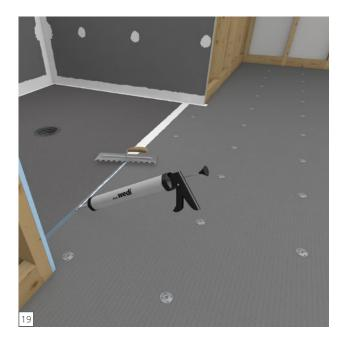
Immediately spread flat all excess sealant with a putty knife. All seams and fastener heads are covered with a secondary 10 mm bead of sealant and spread flat. The seams should be covered 25 mm on either side of seam. All fastener/washers are covered with sealant stretching 25 mm over the washer
