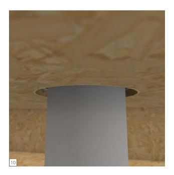
You can then push the Fundo Shower Base including the wedi Drain Unit into the adhesive bed firmly so that the entire Drain Body including adapter is sitting into the DN80 or DN100 Pipe
