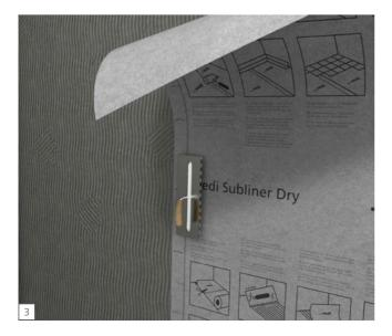
Adhere the wedi Subliner Dry onto the adhesive. Here, air pockets and creases must be avoided.
