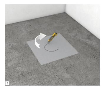
The floor drain area is carefully cut out using a utility knife.
