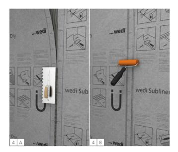
Place the sheets joint to joint or with overlapping joints (the sheets must overlap by approx. 5-10 cm). Any air pockets and creases should be removed.
