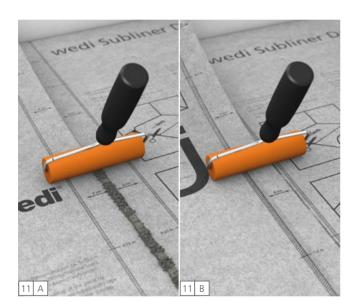
Place the sheets joint to joint or with overlapping joints (the sheets must overlap by minimum 50 mm). Remove any excess adhesive, air pockets and creases using your roller or wooden float. Avoid cross joints.
