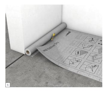
Lay out wedi Subliner Dry and cut to size with a cutter knife or scissors.
