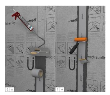
If wedi sealing membranes are butt jointed with wedi Subliner Dry, they are bonded to one another and sealed at the joint with wedi 620 sealant. wedi 620 is applied to the full surface of the sealing membrane without bubbles and with correct coverage. The sealant is applied to both sides of the sealing membrane joint area with a fine-toothed trowel or similar, approx. 10 mm above the edge of the sealing tape (or moulded part or sealing membrane).
