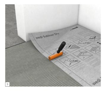
Using a rubber roller or wooden board/float, press the full surface of wedi Subliner Dry onto the surface with the printed side facing upwards. Around the drain, the sealing membrane is adhered into the recently applied sealant wedi 620.
