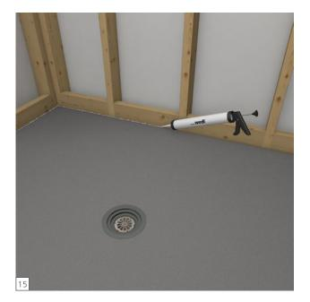
Set up a continuous 10 mm bead of wedi 610 adhesive sealant along the pans channel on the outer perimeter and only in areas where you can immediately install a building board into the fresh sealant.
