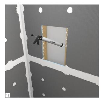
wedi Niches are installed in a cut out in the wedi wall and attached with it's flange right into the center of 450 mm studs. wedi 610 adhesive sealant is set along the connection of wall to niche.
