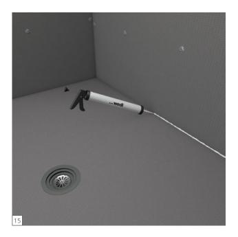
Apply continuous 10 mm beads of sealant between all connections of boards and install with thigthly butted seams. Excess sealant must be spread flat with a putty knife. All seams and fastener heads in the assembly are covered with a secondary 10 mm bead of sealant and spread flat. The seams should be covered 25 mm on either side of seam. All fastener/washers are covered with sealant stretching 25 mm over the washer edges.
