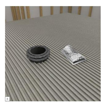
Apply the wedi provided safe Lubricant to the black rubber ring adapter
